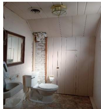
Scott Duncan's handicapped accessible work in progress.
